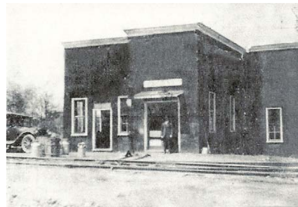
This is the Interurban Dispatching Building that was located near the Hendersonville Presbyterian Church.
