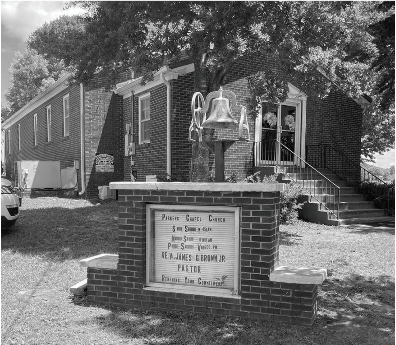
Parker's Chapel Missionary Baptist Church, built in 1956, is rooted to the 150-plus-year-old community it serves
