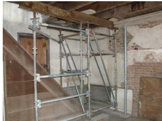
Photo by Rick Hendrix Hawthorn Hill Plaster and borders were repaired.
